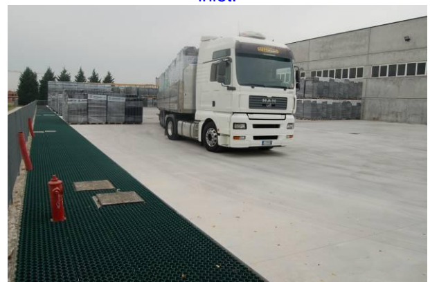
Fig. 5 Finished loading area with R.C. slab
