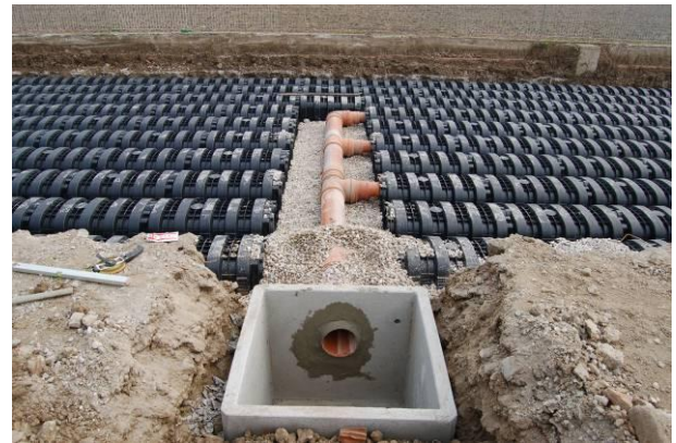
Fig. 3 Detail of the inspection manhole before the main inlet.
