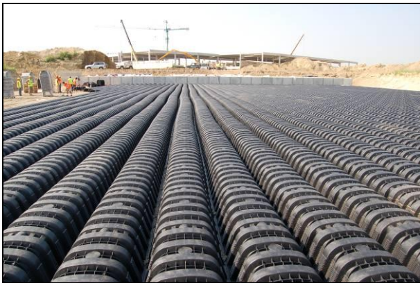
Fig. 2 Installation of the Drening chambers
