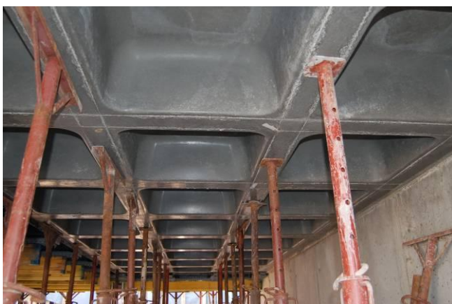
Fig. 4 Concrete after stripping
