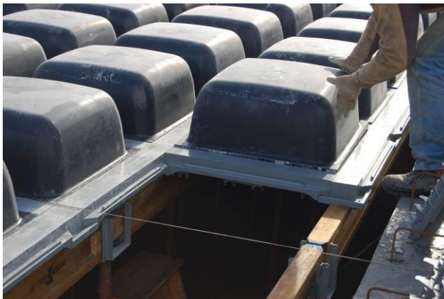
Fig. 2 Ease of assembly and low form weight
