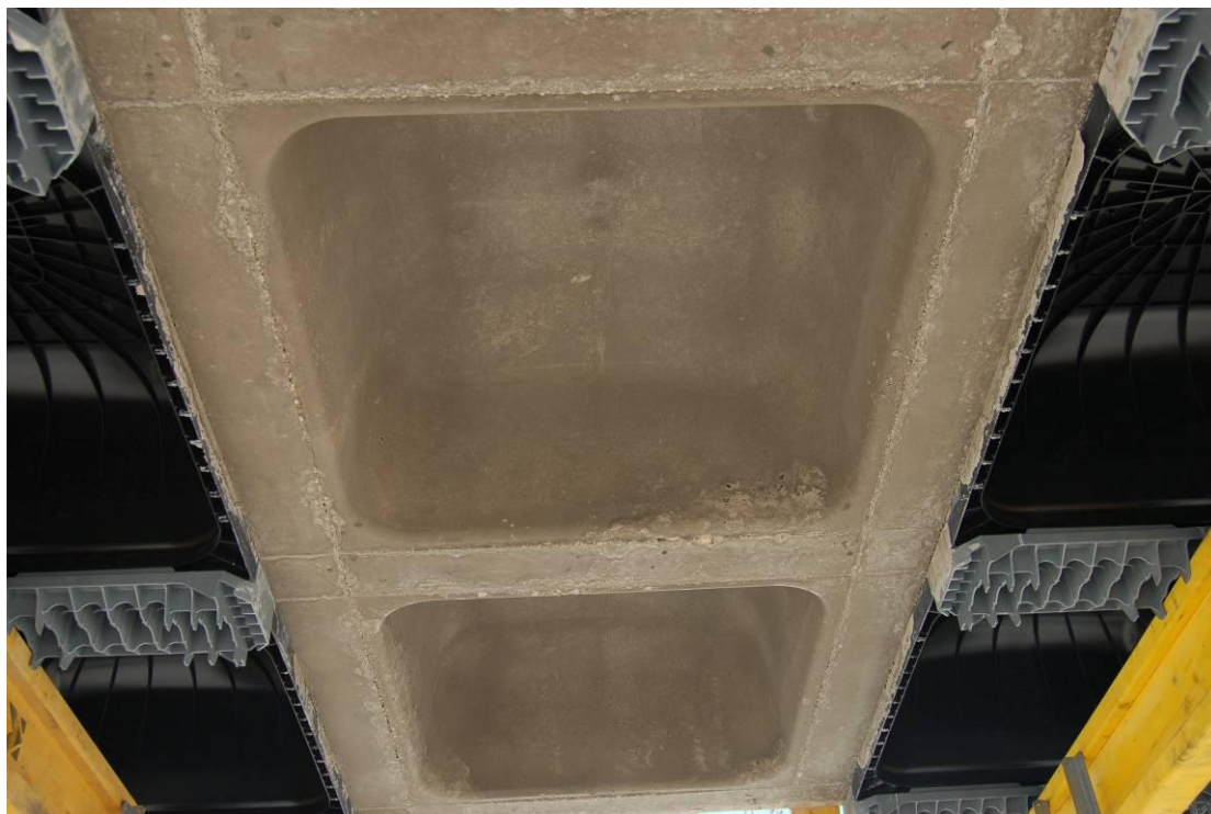
Fig. 4 Detail of the concrete as-is after stripping
