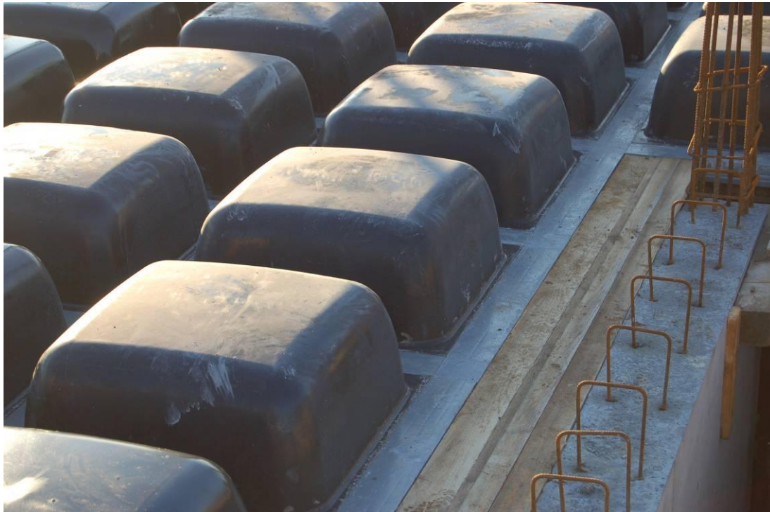
Fig. 3 Detail of lateral compensation with timber plank
