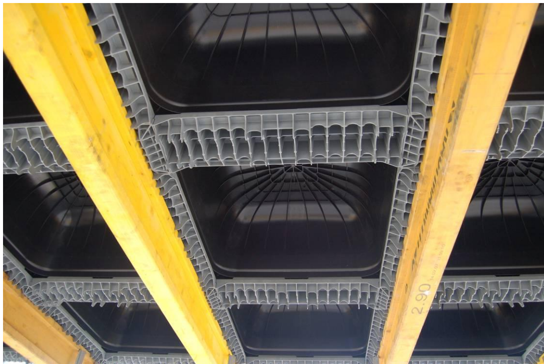
Fig. 2 View from below of the Skydome system
