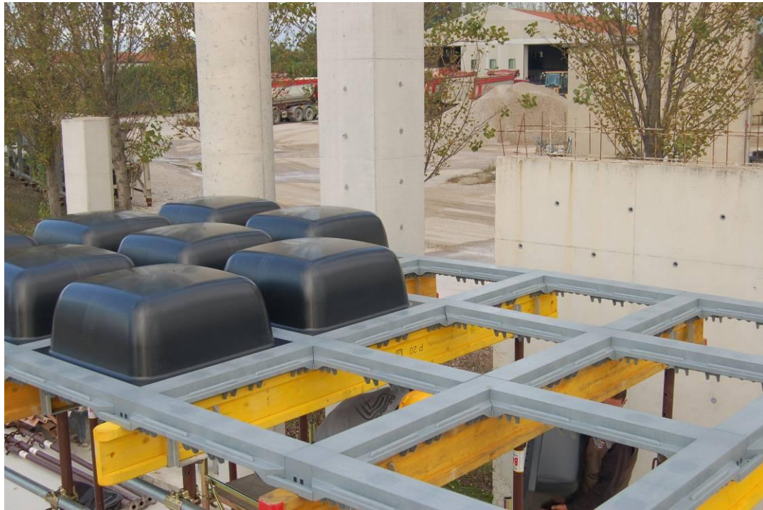
Fig. 1 Placing the Skydome elements
