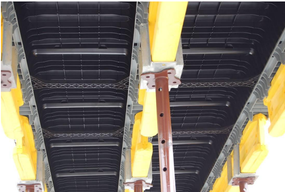
View from below of the forming system
