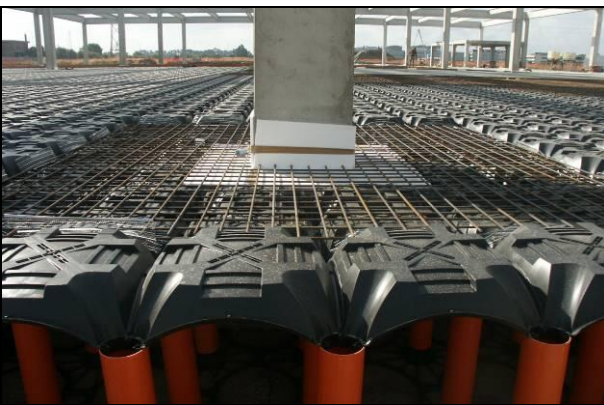
Fig. 3 Slab thickening around the columns
