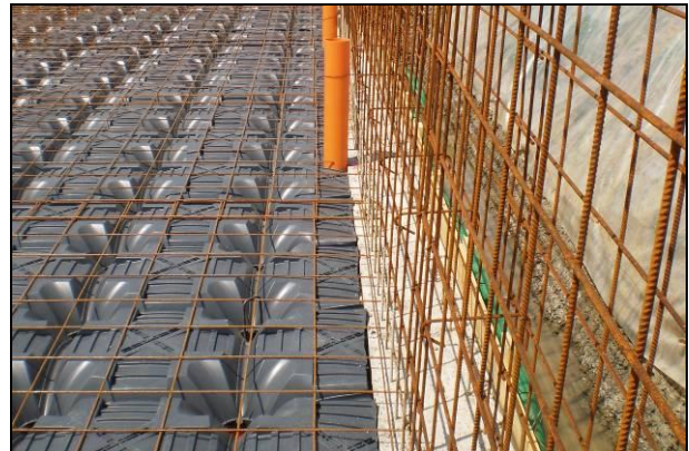
Fig. 2 Detail of the trimmed forms close to perimeter wall
