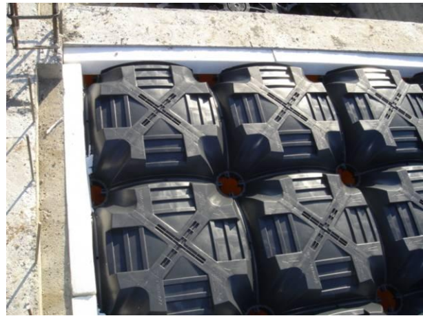
Fig. 2 Detail of the polystyrene compensation strip
