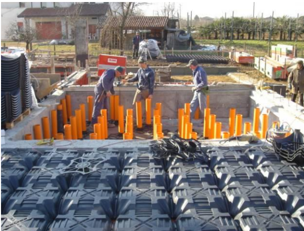
Fig. 1 Installation of Elevetor
