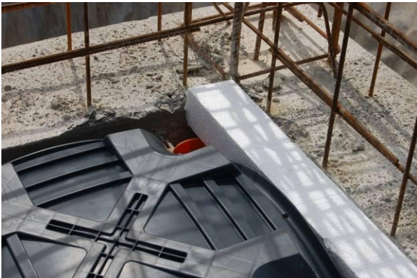
Fig. 3 Detail of the compensation with a strip of polystyrene
