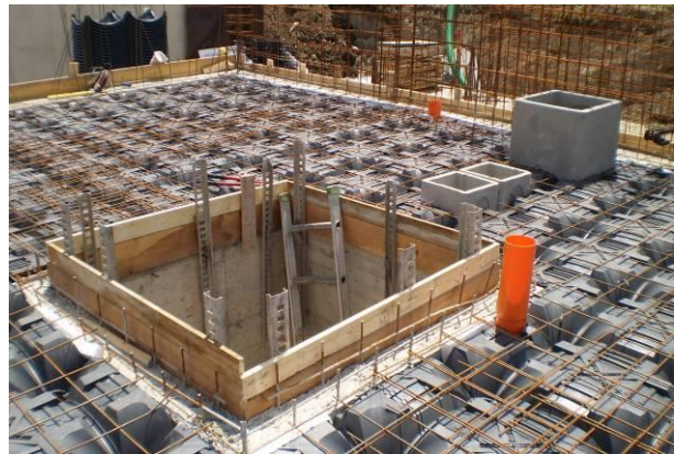
Fig. 2 Detail of the lift shaft
