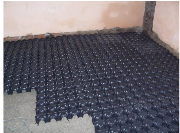
Fig. 2 Laying of Modulo
