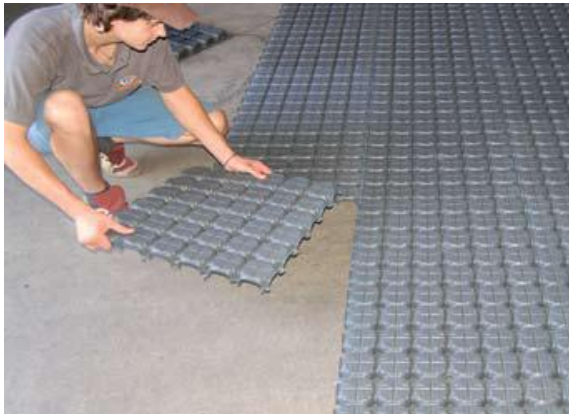
Fig. 1 Installation of Minimodulo
