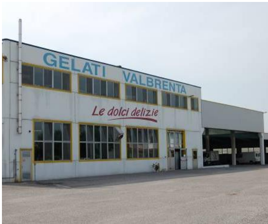
Fig. 1 View of the building from the outside
