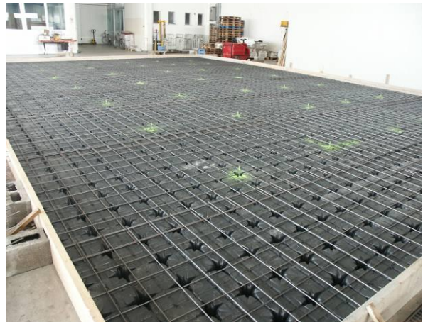
Fig. 2 System installed and ready for the pour
