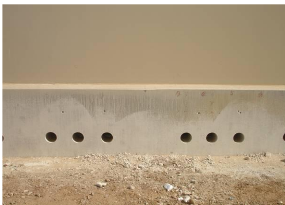
Fig. 3 Detail of the ventilation holes
