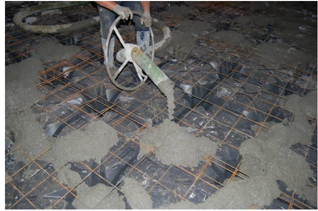
Fig. 2 Initial pour phase (the pockets must be filled first)
