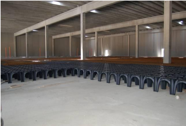
Fig. 1 Installation of Modulo and armature
