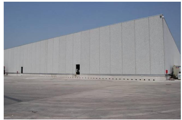
Fig. 4 Building seen from outside
