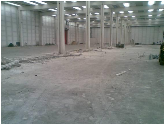
Fig. 1 Existing warehouse floor
