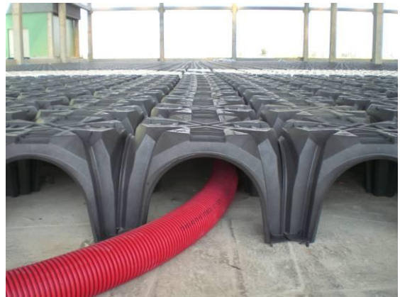
Fig. 2 Installation of Modulo and piping
