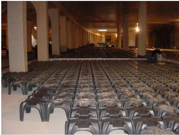
Fig. 1 Installation of Modulo
