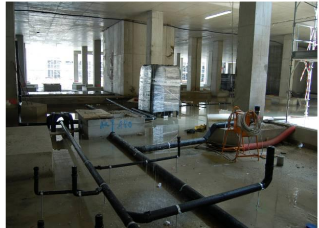
Fig. 2 Installation of the plumbing
