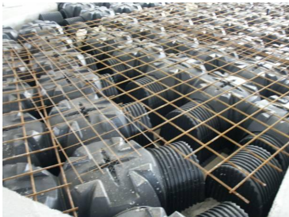
Fig. 3 Detail of corner formed with the aid of Geoblock
