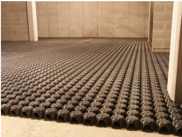
Fig. 1 Modulo installed on groundslab
