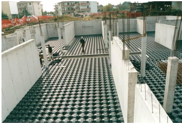
Fig. 1 Modulo installed on groundslab
