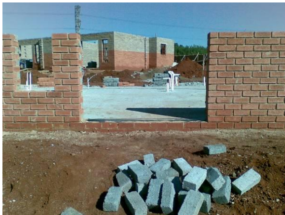
Fig. 3 Building in progress
