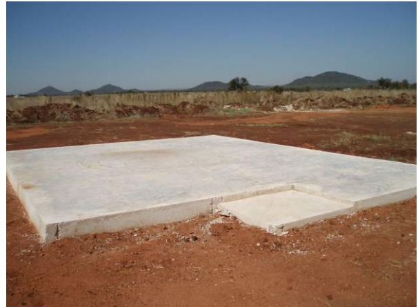
Fig. 2 Finished groundslab
