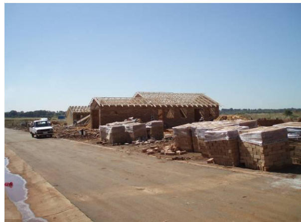
Fig. 4 House in construction
