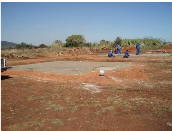
Fig. 3 Finished groundslab
