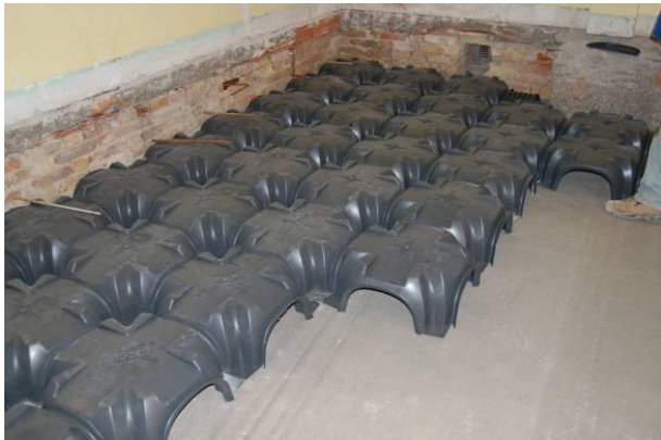
Fig. 1 Installation of Modulo
