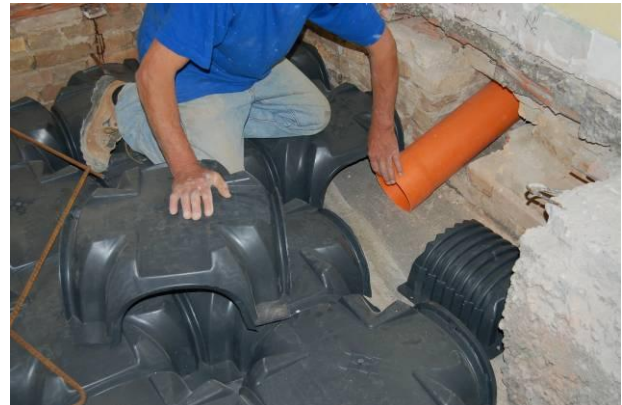
Fig. 2 Detail of ventilation piping
