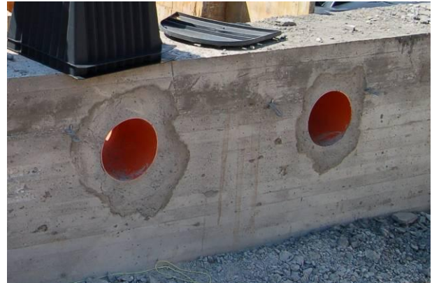
Fig. 2 Detail of ventilation holes
