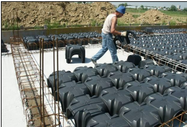
Fig. 1 Installation of Modulo
