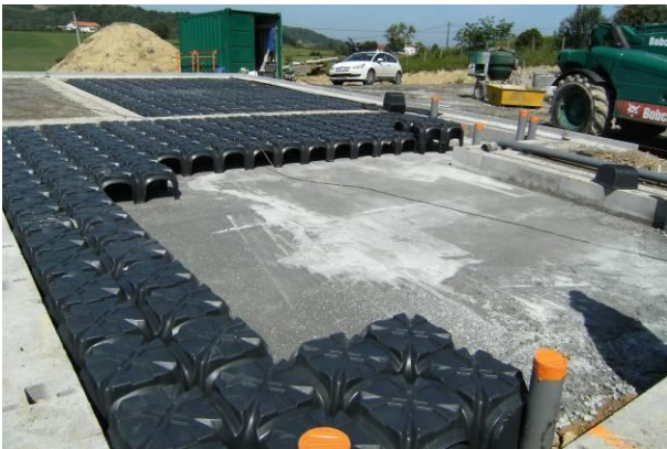
Fig. 1 Installation of Modulo
