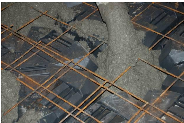
Fig. 3 Initial pour phase (the pockets must be filled first)
