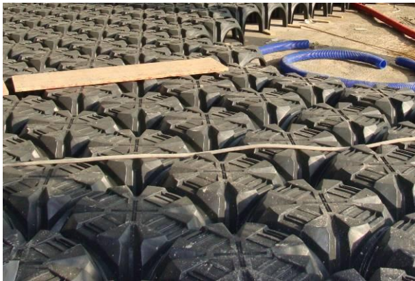
Fig. 1 Installation of Modulo
