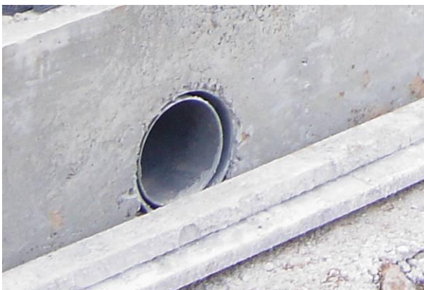
Fig. 3 Detail of ventilation hole
