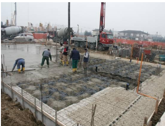
Fig. 3 Initial pour phase (the pockets must be filled first)
