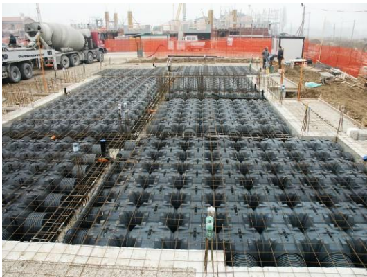
Fig. 1 Installation of Modulo
