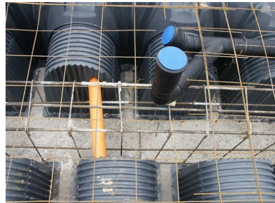
Fig. 2 Detail of ventilation connection
