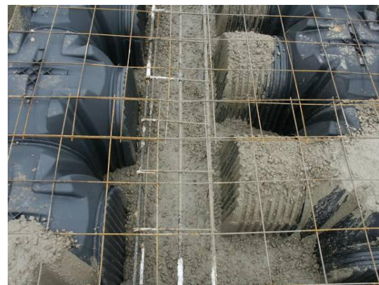
Fig. 4 Detail of monolithic foundation pour – ground beam
