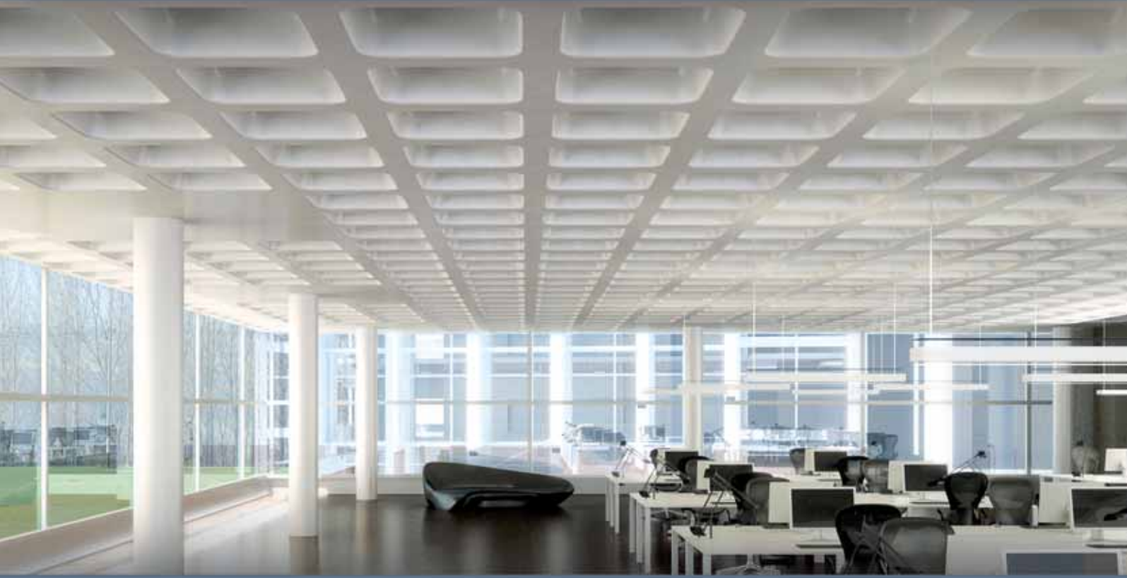
The lightweight waffle slab formwork
